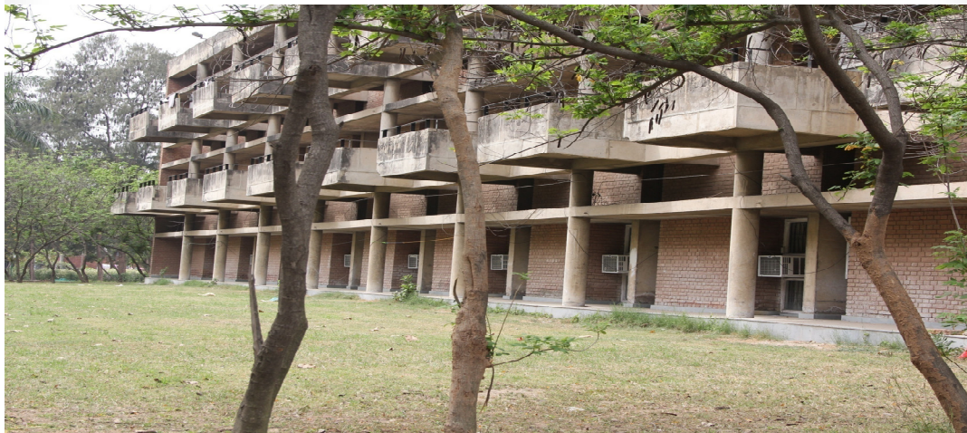
AIR CONDITIONERS INSTALLED IN FACULTY HOUSE
