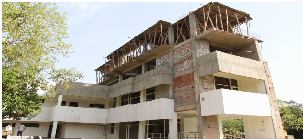
Expansion of PU Guest House
